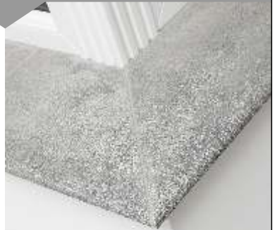
Example of a finished mitre corner
